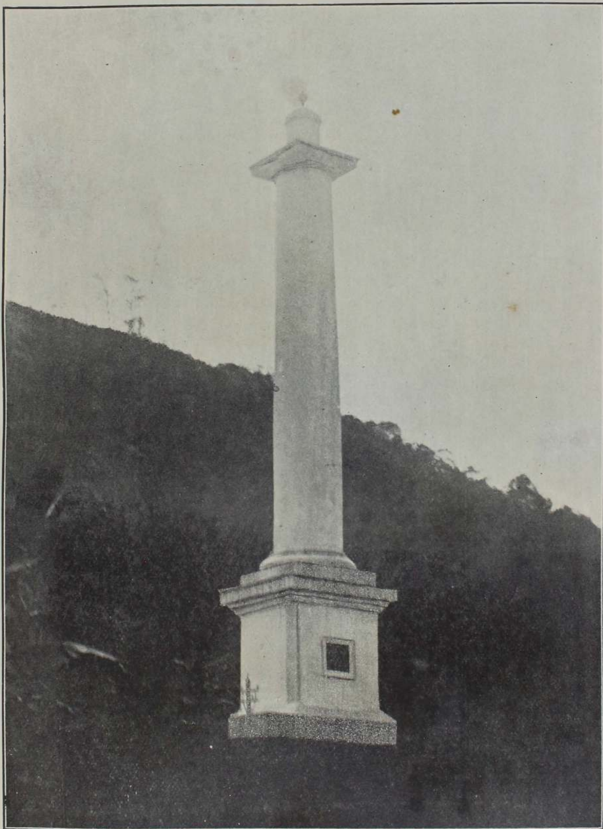
MONUMENT AT KADUGANNAWA Erected to the Memory of CAPTAIN W. F. DAWSON Commanding Royal Engineers Ceylon 1825 - 1829.
