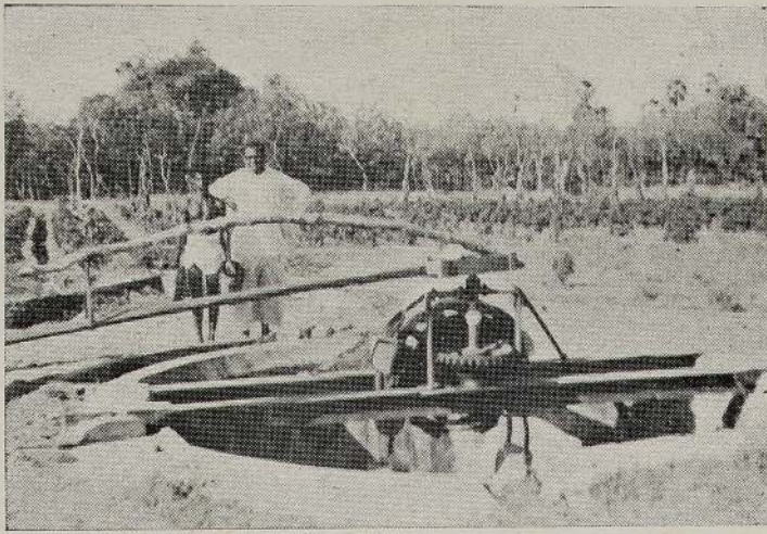
PHOTO 1.—Bullock operated water lift on well.
