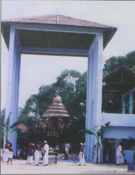
Newly built Ther shed
