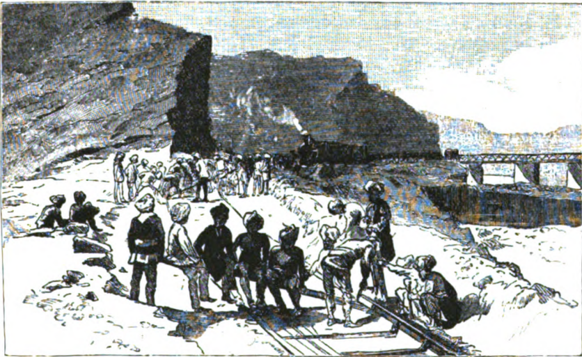
TRACK-LAYING NEAR BHOPAL.
