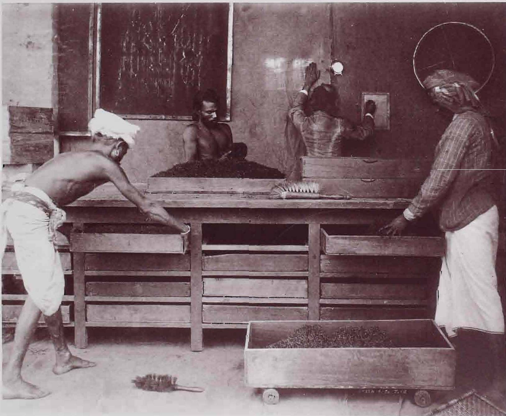
Green leaf is converted into black tea in five steps, withering, rolling, fermenting, firing and sifting. On these two pages are scenes of early tea manufacture. Above, the manufacture takes place in an old coffee store c.1885. Those were the days when the rolling of the leaf was done by hand and firing was done by placing trays of rolled leaf over pits of glowing charcoal. On left, a day's fired leaf is examined by the men. On facing page, top, the beginnings of mechanisation, but still in an old coffee store. The two women sort the fired leaf laid out on the floor. On facing page, bottom, fired leaf is spread by one man, gathered by another and sieved by the third. And on page 50, more sifting, using a sieve as well as the traditional South Indian winnows.
