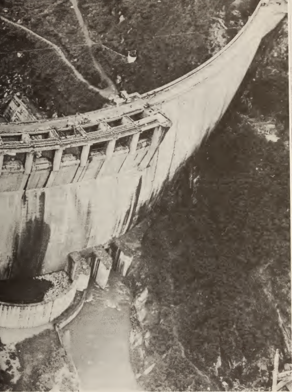
Victoria Dam approaches completion, Accelerated Mahaweli Program Courtesy Embassy of Sri Lanka, Washington
