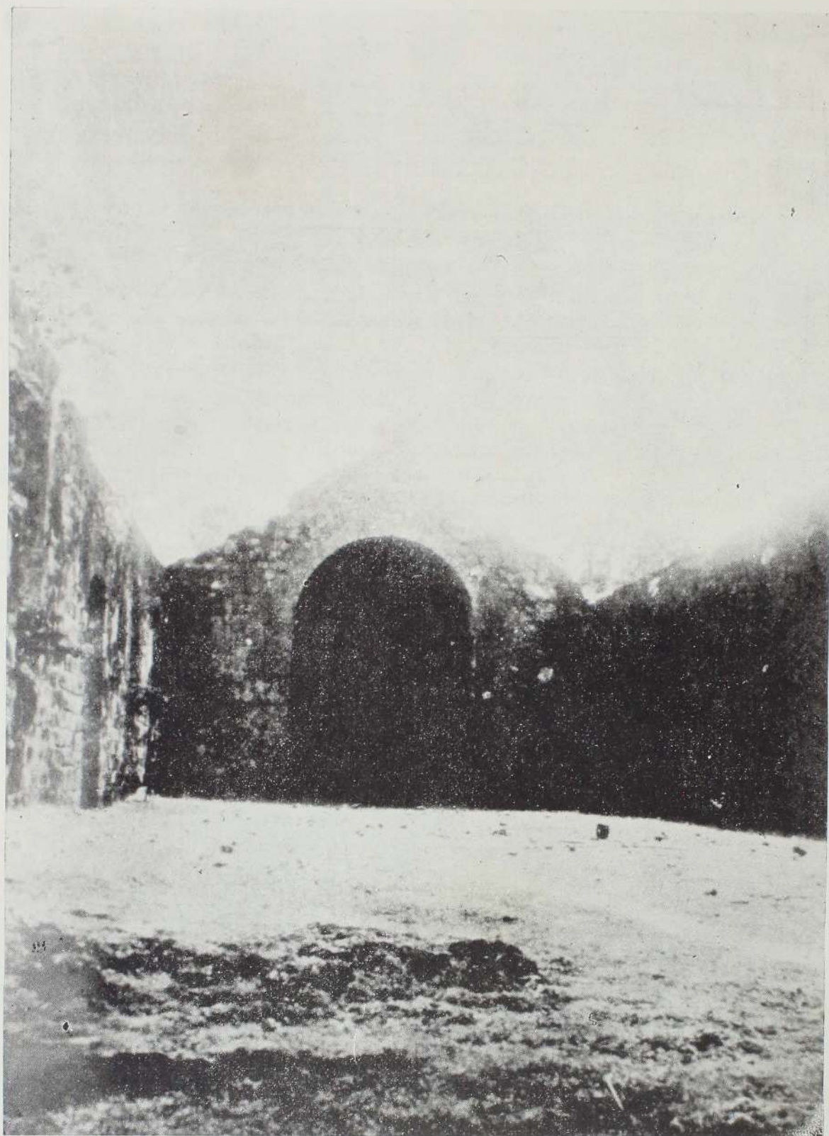
What is left of the Church at Chankanai. It is still possible to trace a nave, a chancel and side aisles. The chancel built in the form of a stone-worked vault, is ascribed to be the only example of its type in Ceylon.
