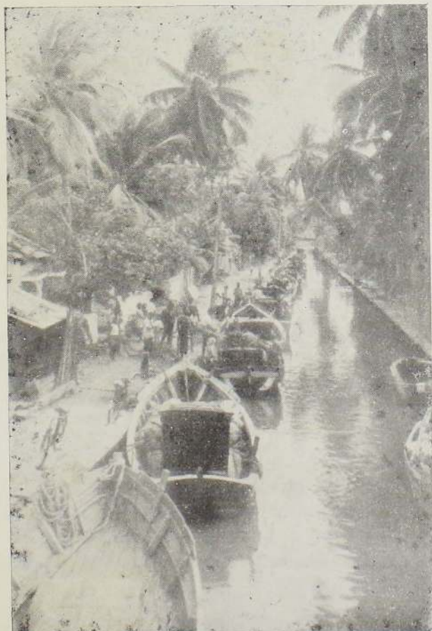
Sections of the old Dutch Canal through Negombo. The top illustration also shows the type of barge (provided with a thatched roof) which the Dutch introduced to Ceylon for use on their Canals. It is called locally : “ padda boat ” and was towed using a tow-path on the bank or poled or sailed.
