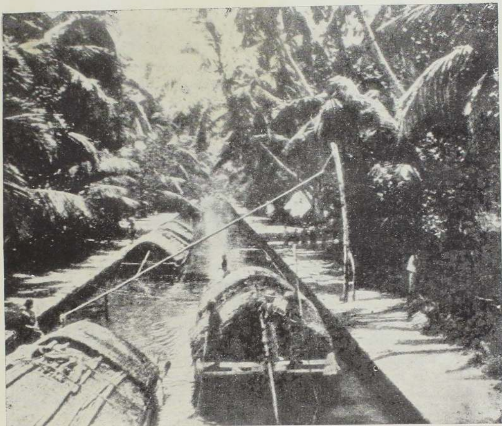
Sections of the old Dutch Canal through Negombo. The top illustration also shows the type of barge (provided with a thatched roof) which the Dutch introduced to Ceylon for use on their Canals. It is called locally : “ padda boat ” and was towed using a tow-path on the bank or poled or sailed.
