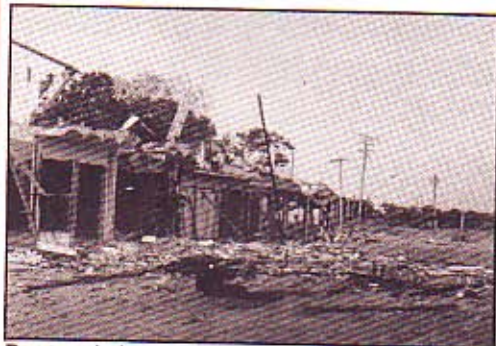
Damaged shops - near market in Kilinochchi.
