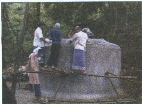
Fig. 3.15 : Building of rain water tanks
