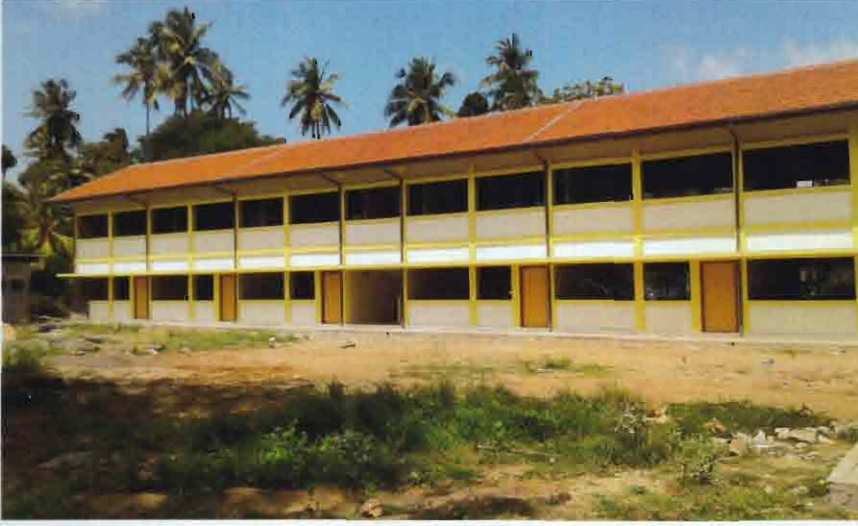
New Classrooms for Primary school
