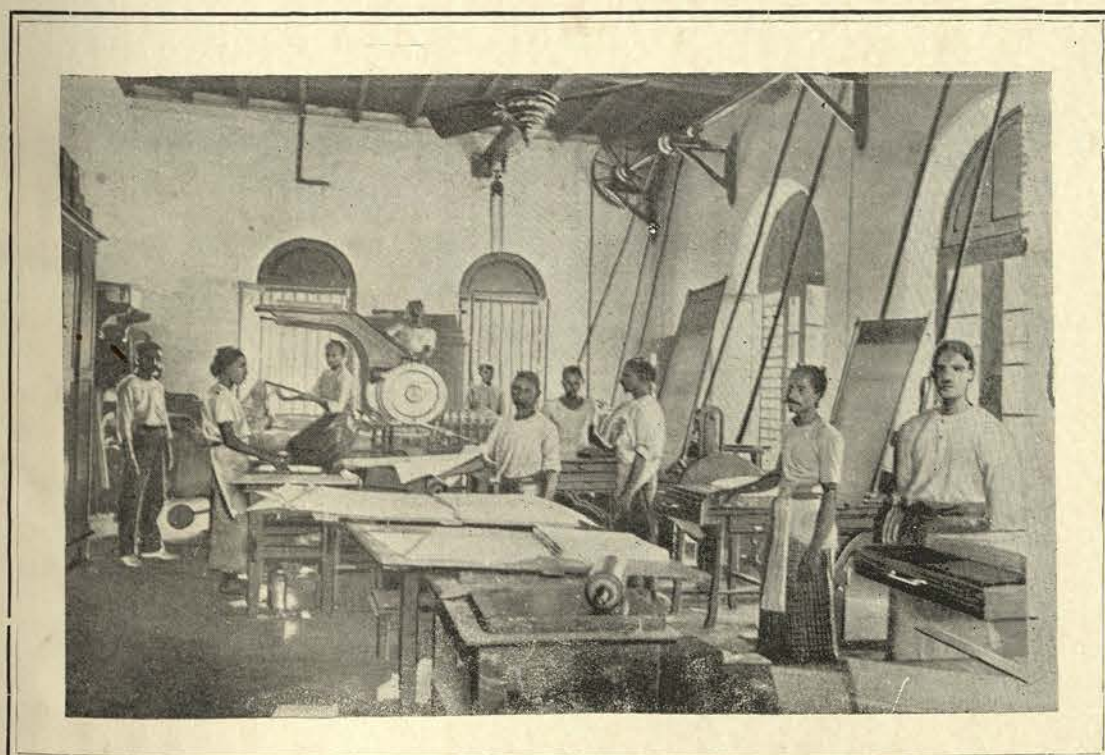
Lithographic Printing Room on the Ground Floor, showing the three Presses and one Machine now in use.
